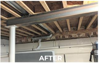
Provided the Structural Repair Calculations and executed the fix by replacing old roof joists & wooden beam with new joists & steel beam respectively
